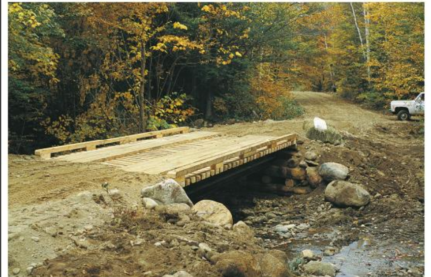
A permanent bridge.
