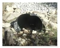
Completed culvert showing streambed material (rocks and sediment) and riprap added.
