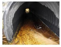
Culvert spans the entire stream width, is embedded below grade, and contains streambed material.
