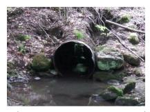
Culvert is too narrow causing pool at inlet. Water backs up during high flow, leading to erosion around culvert and washouts.
