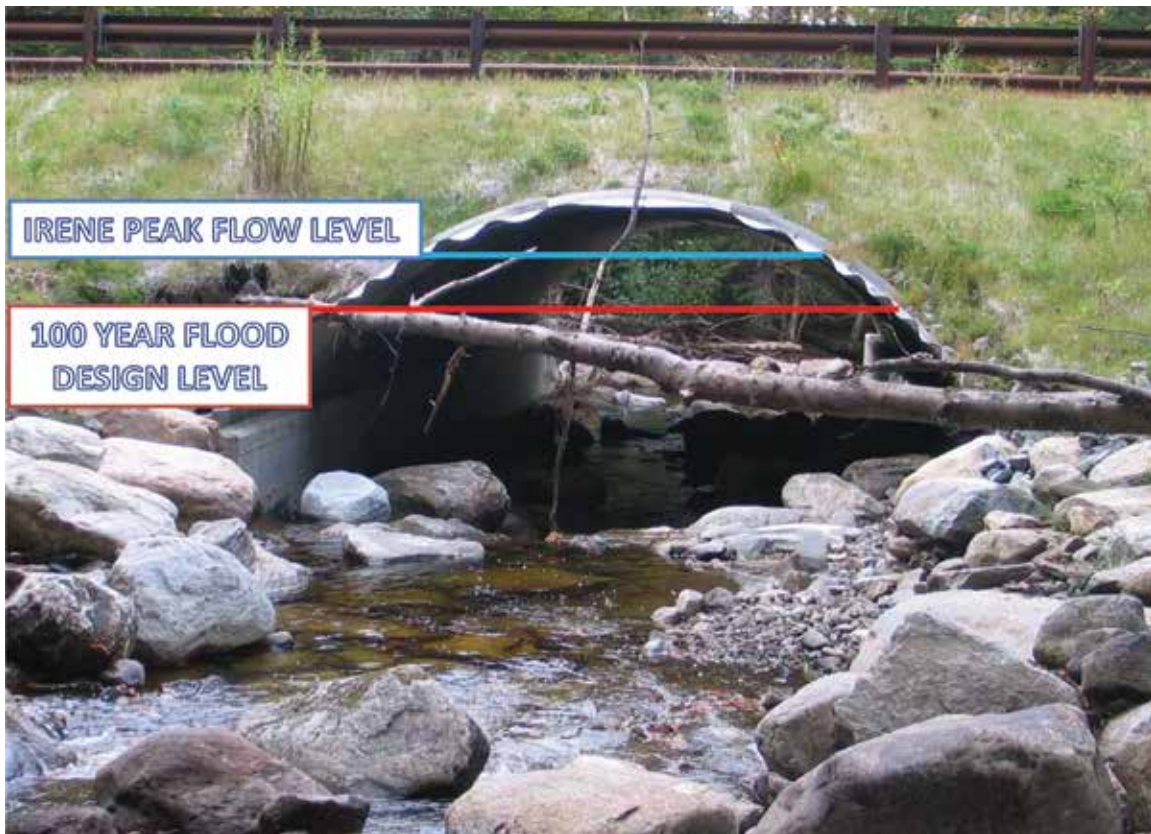
Figure 5. Stream simulation design culvert at Jenny Coolidge Brook, installed in June 2010, showing height of 100-year design discharge in red and height of Tropical Storm Irene flood level in blue. Photo credit: Brian Austin, Green Mountain National Forest.
